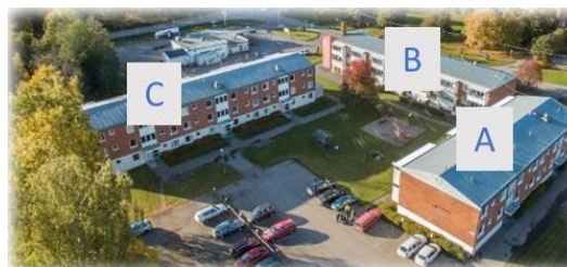
Fig. 1: Three buildings in the cluster for renovation in Ludvika, Sweden.
